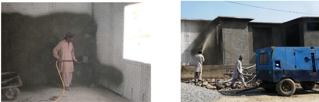
Figure 08:Applying Concrete
