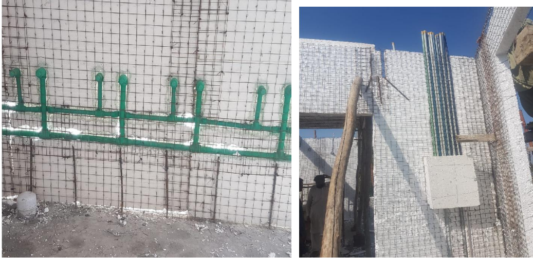
Figure 07: Installation of utilities before concreting
