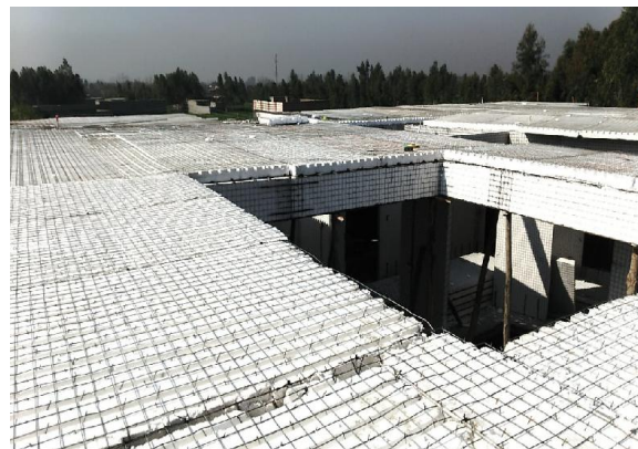
Figure 06: Placed Slab panels on wall panels
