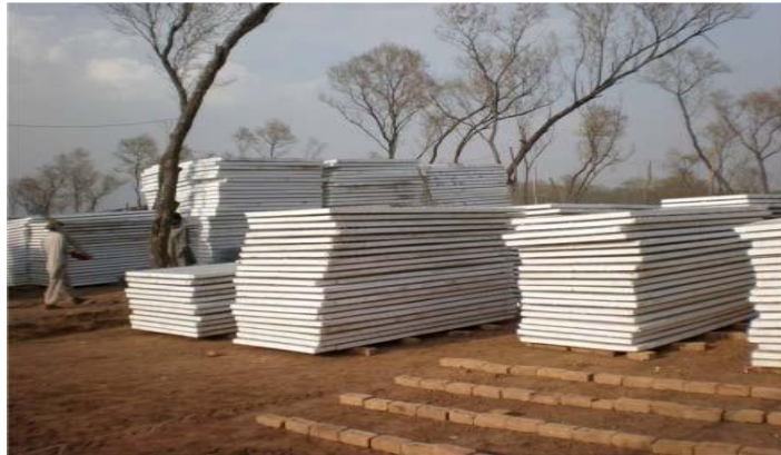
Figure 04: Transportation of panel to site
