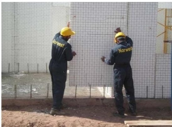
Figure 05 : Placing panels in dowels
