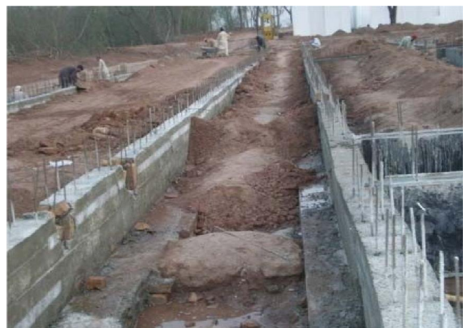
Figure 03: Leaving dowels in foundation
